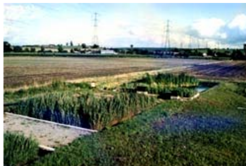
Fig.7 Horizontal reed bed treatment system serving a Population of approximately 15 persons.
