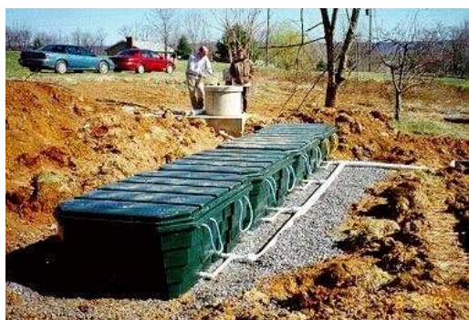
Fig 11 Eight module Puraflo™ system
