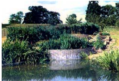
Fig.6 Attractive horizontal and vertical reed bed sewage treatment system followed by a pond (foreground)
